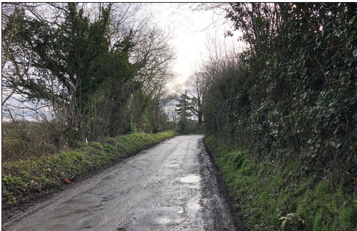
Figure 2.5 The Rathmullan Road runs alongside the northern, eastern and southern boundaries of the subject site.
